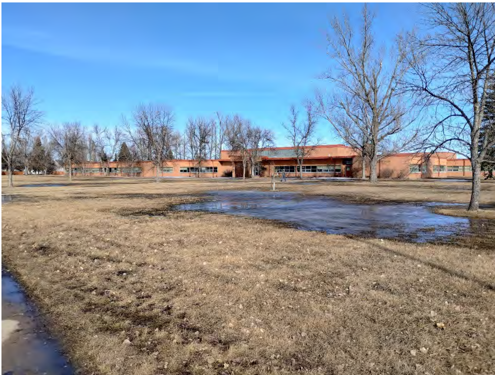
Figure 6. Overview of the Eielson School, west façade, view to the east-northeast.
