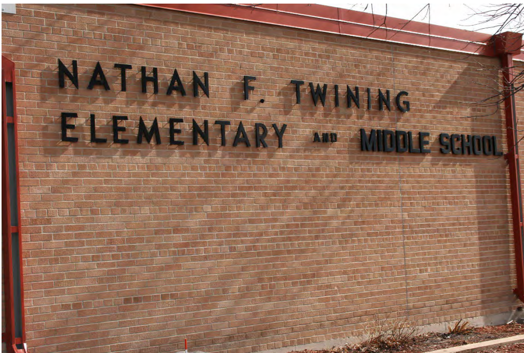
Figure 41. Twining School lettering, view to the east-southeast.
