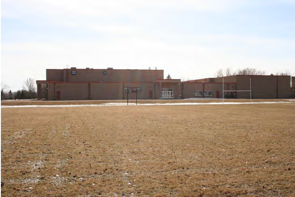
Figure 30. View of Twining School's north side looking south. Left and center: 2003 addition; far right: 1964 addition.
