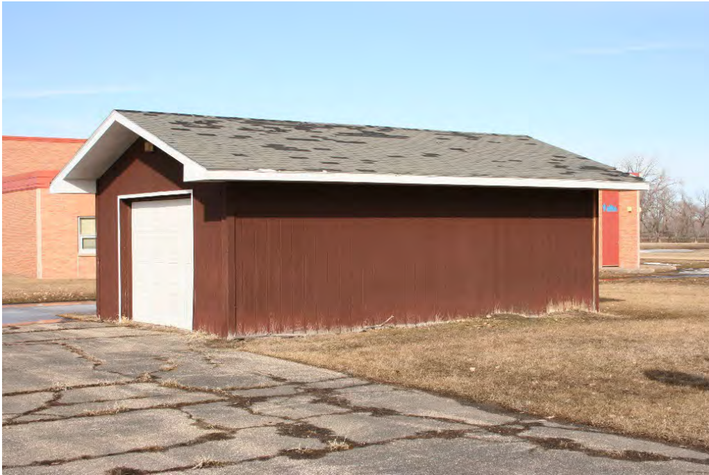
Figure 19. Modern detached garage building at Eielson School site, view to the northeast.
