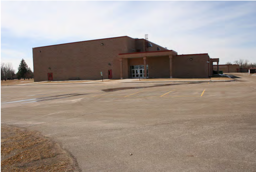
Figure 28. View of Twining School's east side (2003 addition) looking west-southwest.
