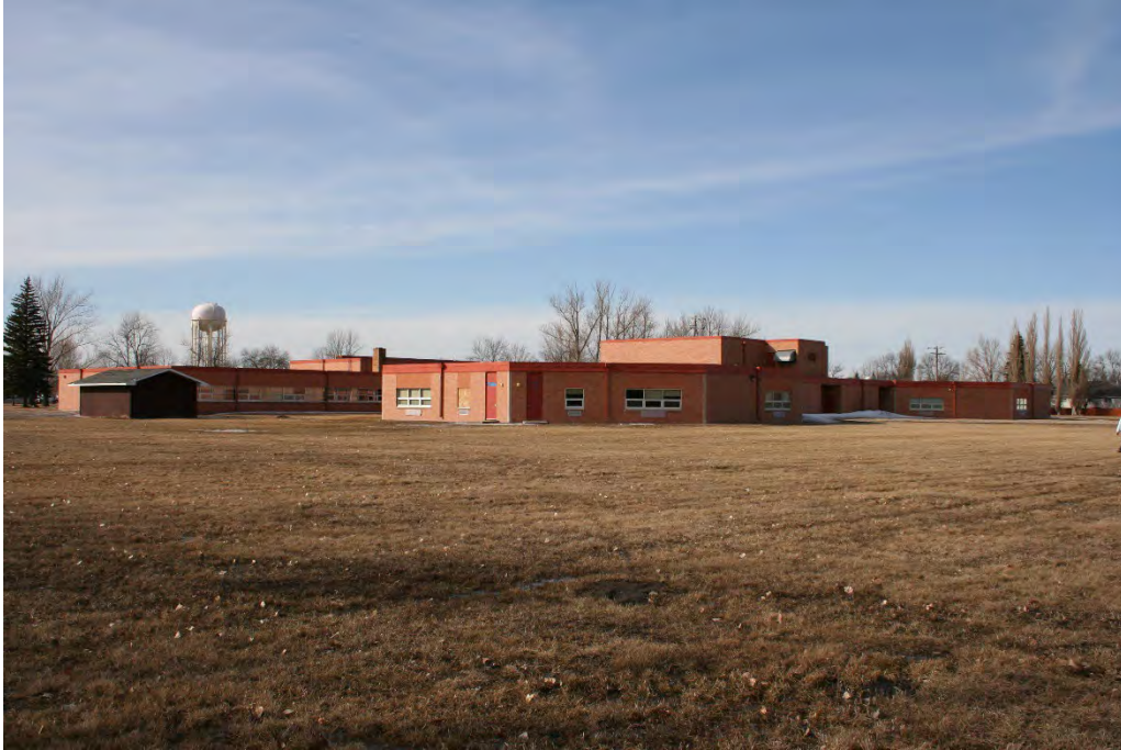
Figure 13. Overview of the Eielson School's southeast corner: octagonal addition (foreground) with original construction (background left), view to the northwest.
