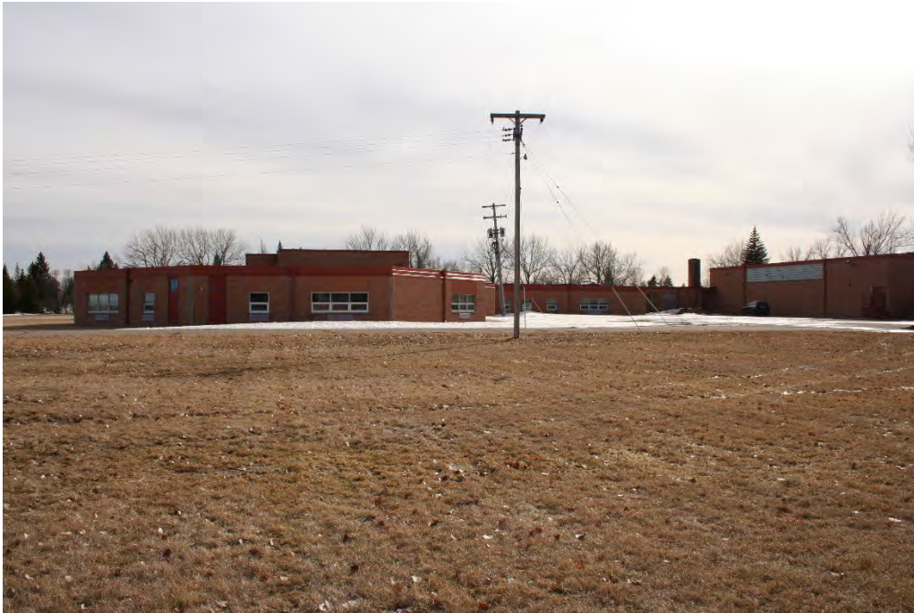
Figure 15. Overview of the Eielson School's northwest corner: octagonal addition (left), original construction (right), view to the south.
