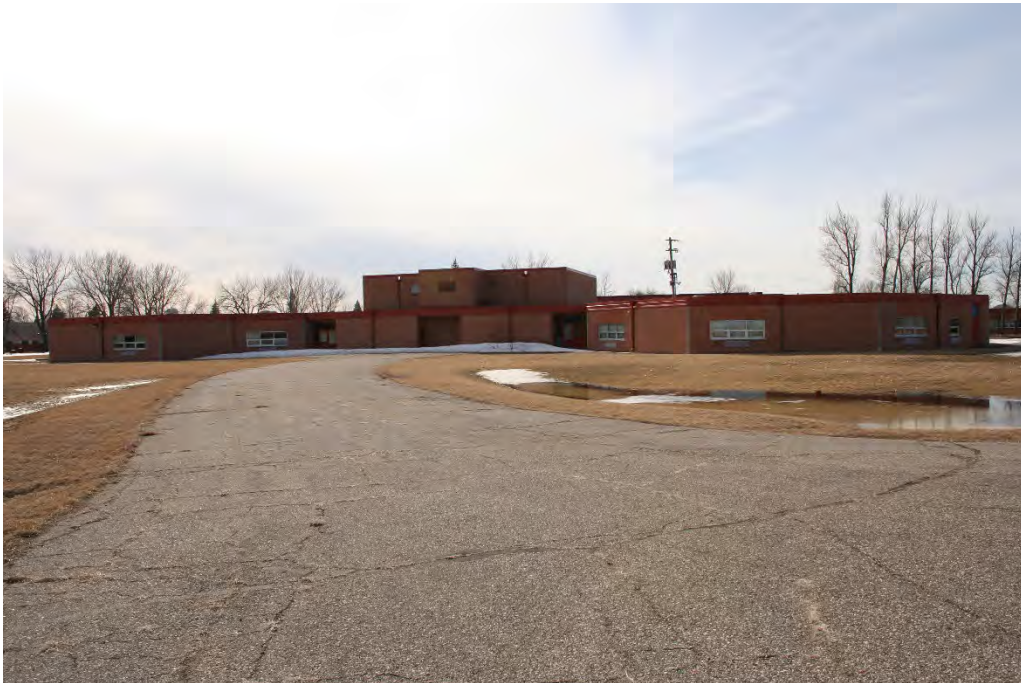
Figure 14. Overview of the Eielson School's east façade/addition, looking west-southwest.
