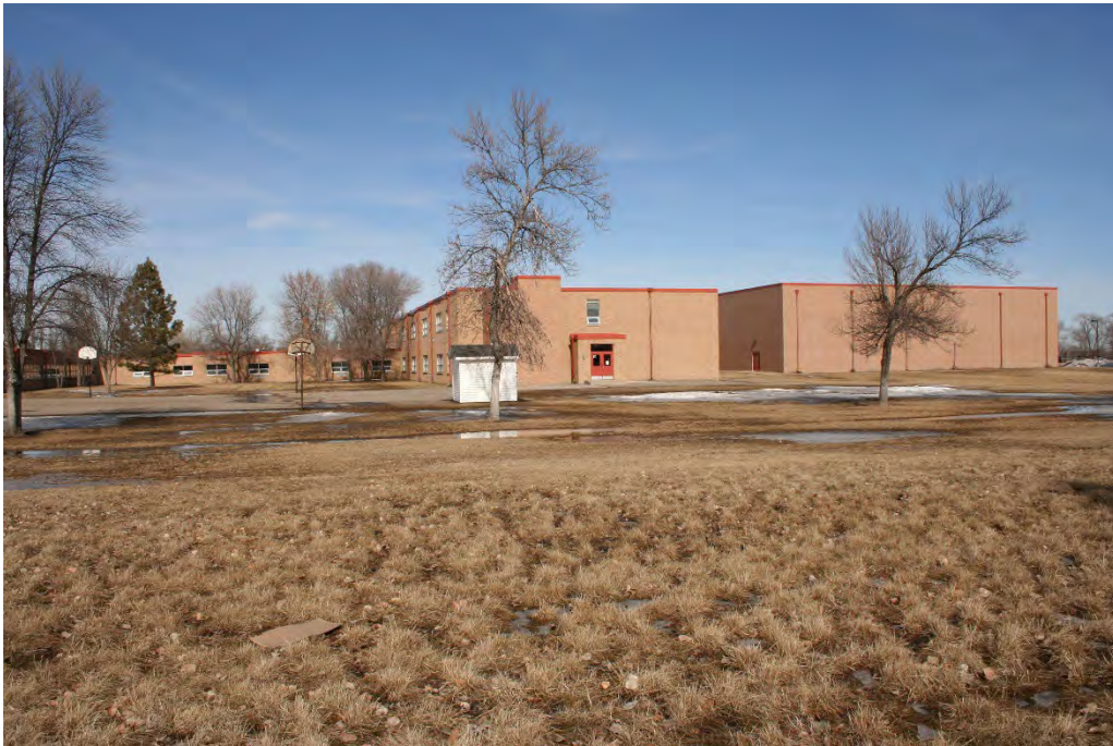
Figure 25. View of Twining School's south side looking north. Left and center: 1964 addition; far right: 2003 addition.
