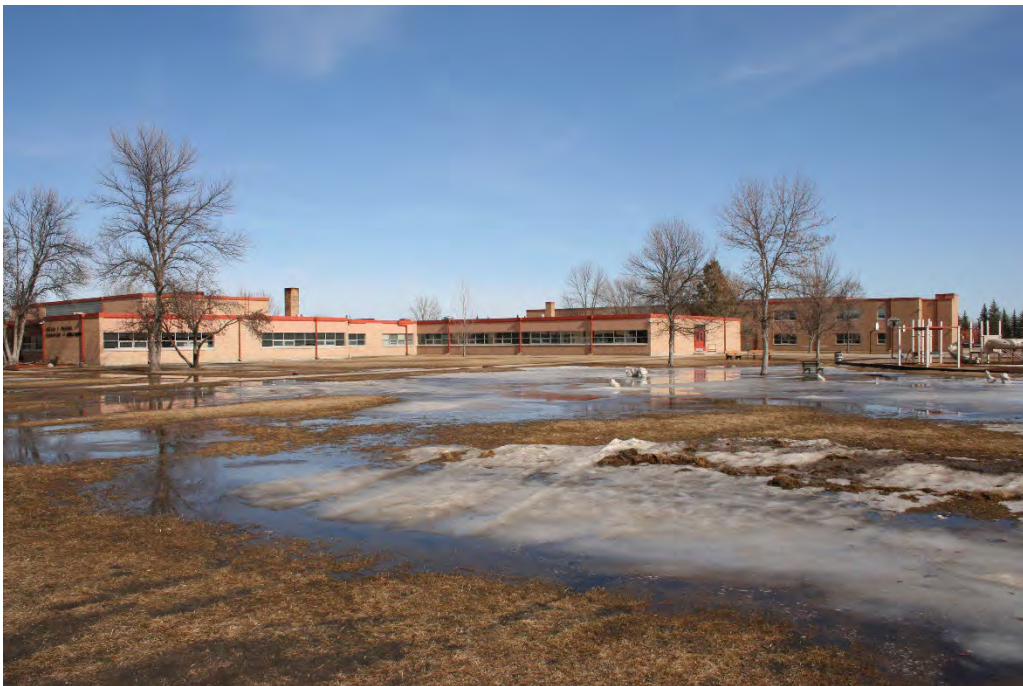
Figure 23. View of Twining School's southwest side looking northeast. Left and center: original 1962 school; background right: 1964 addition.
