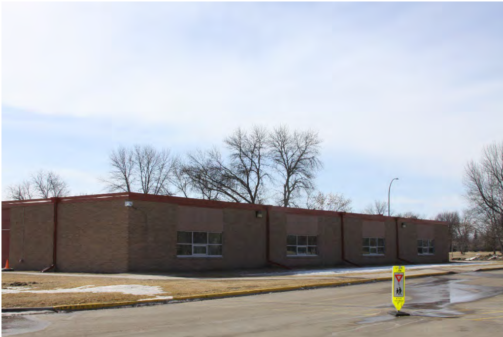
Figure 35. View of Twining School's northeast side (1966 addition) looking southwest.
