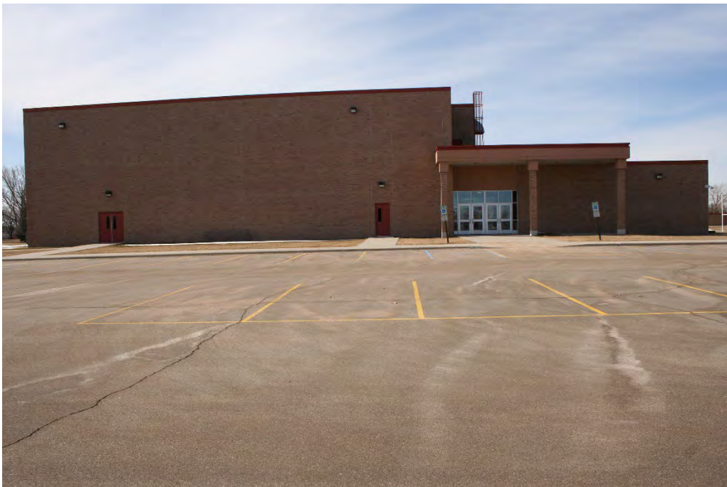
Figure 27. View of Twining School's east side (2003 addition) looking west.
