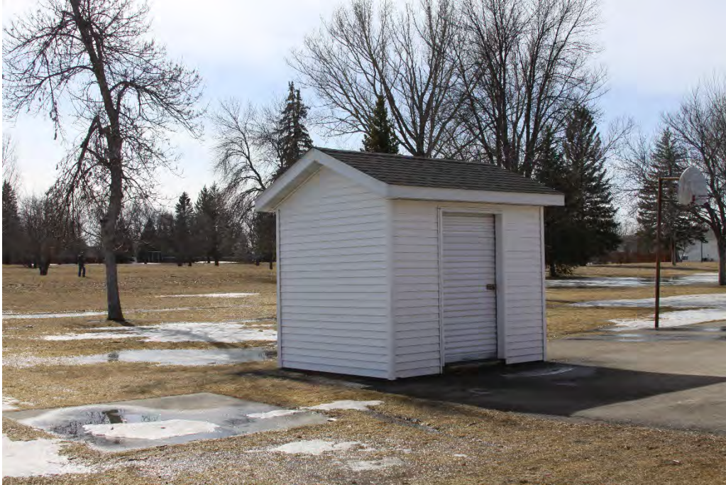
Figure 46. Modern shed at the Twining School site, view to the southwest.
