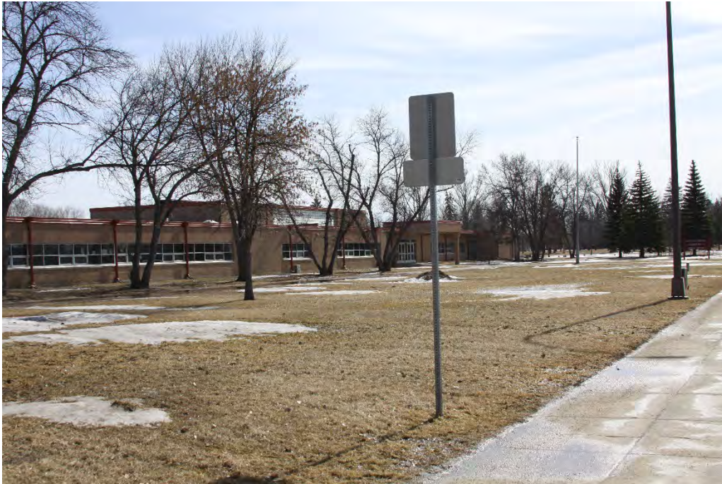
Figure 38. View of Twining School's west side (original 1962 construction) looking southeast.
