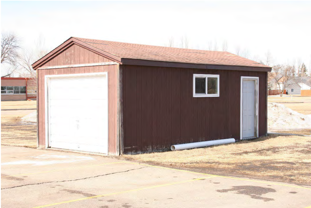
Figure 44. Modern detached garage at the Twining School site, view to the northwest.
