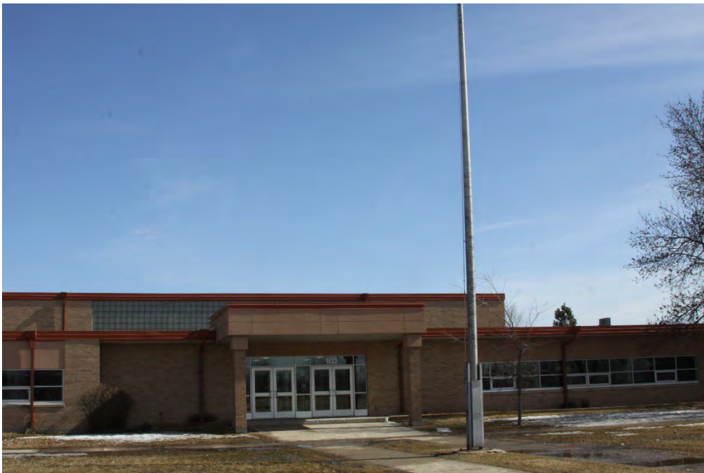
Figure 39. West façade Twining School entry, original 1962 construction, looking east.
