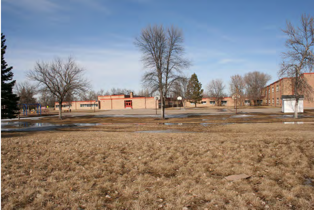
Figure 24. View of Twining School's south side looking north. Left: original 1962 construction; center right and far right: 1964 addition.
