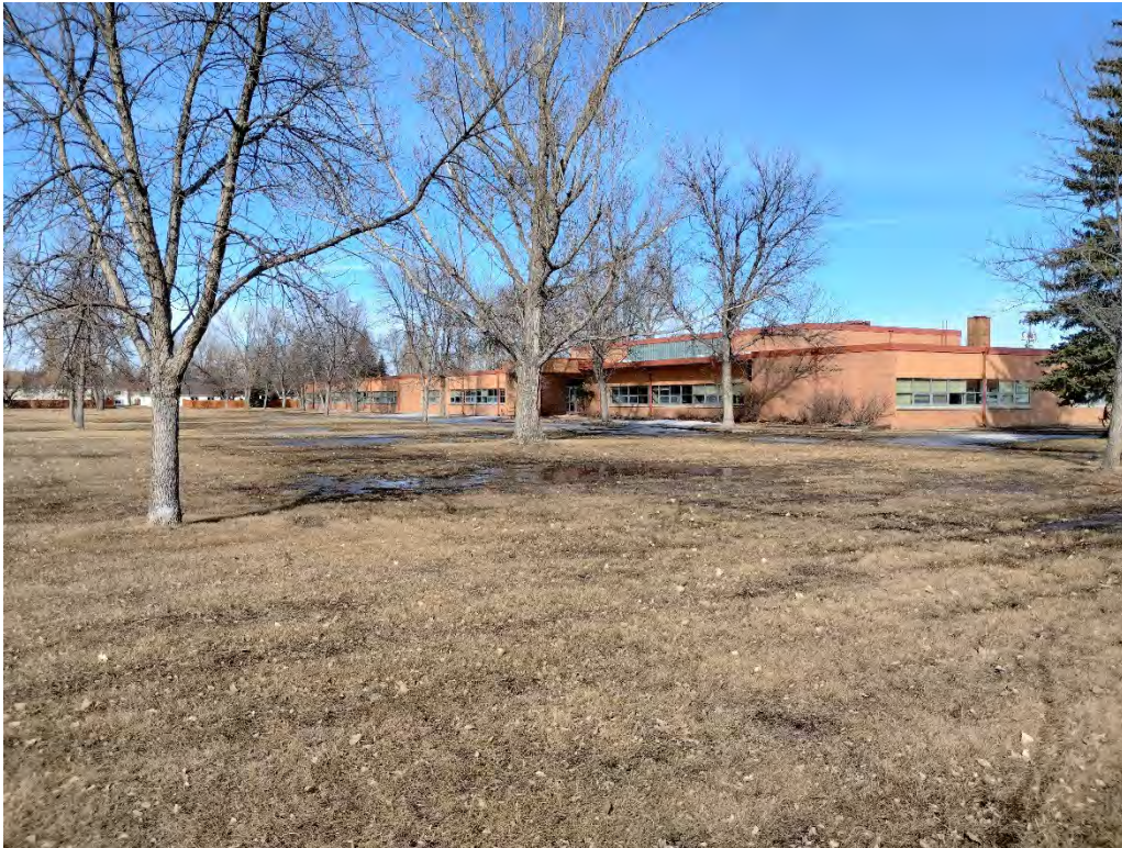
Figure 7. Overview of the Eielson School, southwest corner, view to the northeast.
