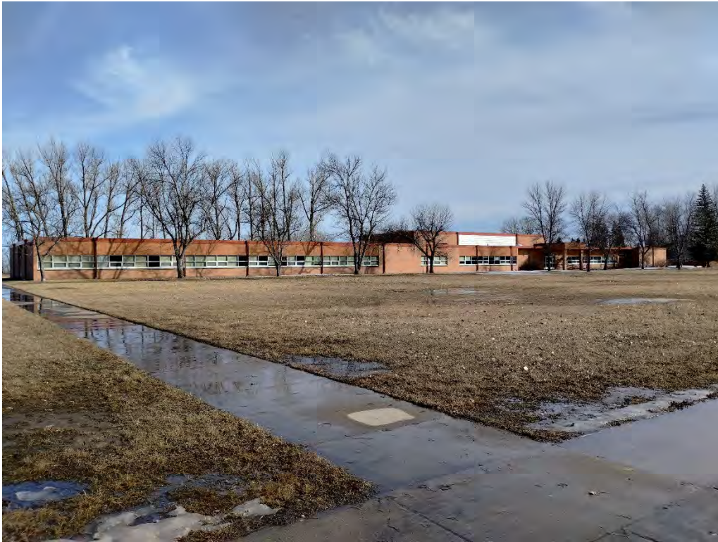
Figure 5. Overview of the Carl Ben Eielson Elementary School, west façade, view to the east-southeast.
