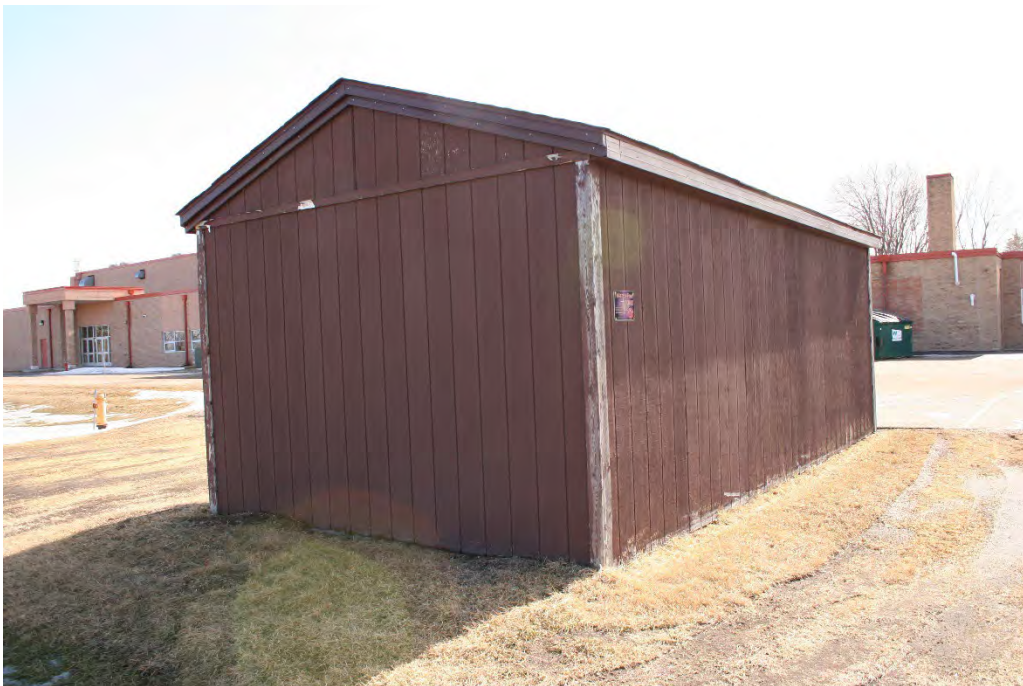
Figure 43. Modern detached garage at the Twining School site, view to the southeast.
